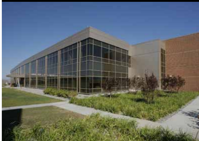
Above | 2010 Building ($10 million and over) | Lydig+Grant, a Joint Venture | Pacific Northwest National Laboratory Physical Sciences Facility
