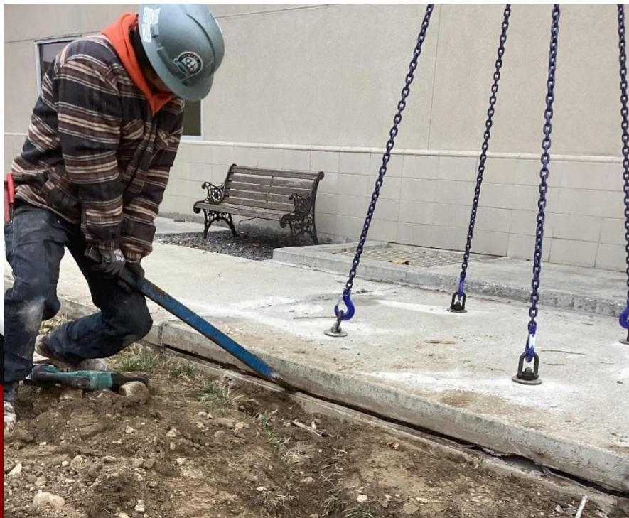
Due to the complexities of the existing conditions multiple precast panels sizes were not finalized until most panel installation was completed. This was a deliberate strategy to avoid waste and rework ensuring a perfect fit for the last few panels.
