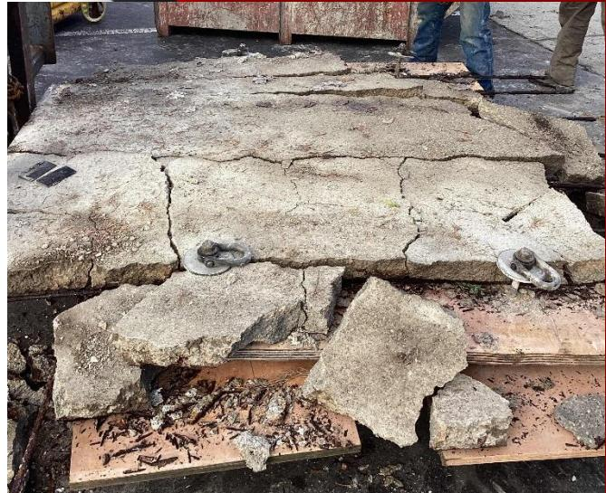
To accomplish this, Clearwater used 1.25" superior-grade plywood as a reinforcement layer and securely anchored picking eyes through the plywood and the existing lid. This distributed the weight evenly and ensured that the fragile panels remained intact during removal. By taking these extra precautions and clear communication between the crew, the team was able to safely lift the deteriorated panels from the tunnel without incident.
